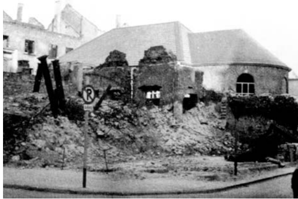
The rebuilt Krefeld Mennonite Church in the midst of the post-war ruins.
