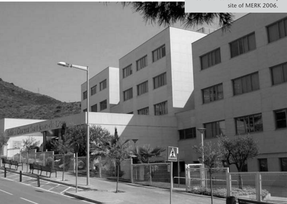
Conference centre in Barcelona, site of MERK 2006.
