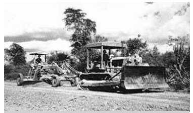
Grading the Transchaco Highway
