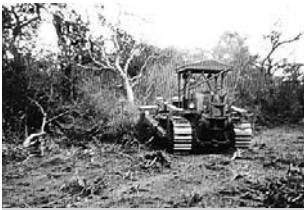
Clearing brush for the Transchaco Highway
